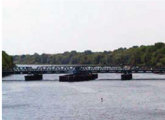
Riverside-Delanco Bridge, the Commission's only swing-span bridge.
