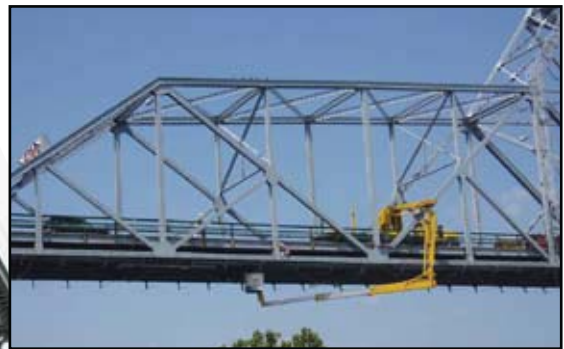
This traveler system will greatly improve the efficiency of inspections and maintenance on the Burlington-Bristol Bridge and save the Commission thousands of dollars. Attached to beams inside the Commission’s Maintenance building, the traveler system will enable maintenance staff and engineers to literally “hang from” the underside of our bridges to inspect and maintain the structures.
