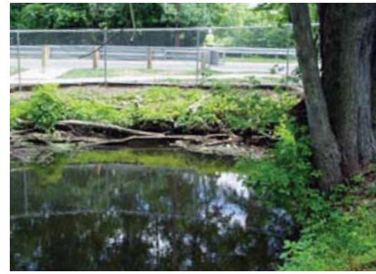
Swede Run Bridge, on County Route 543 in Delran.
