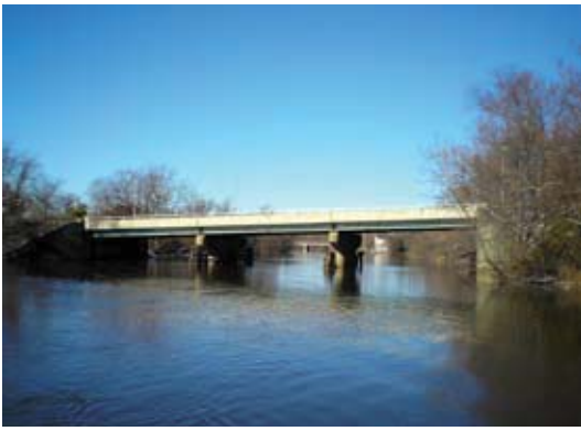
Pompeston Creek Bridge, on County Route 543, in Riverton.
