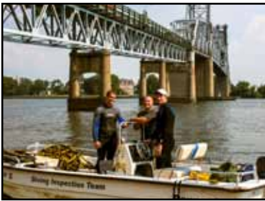
In-depth bridge inspections, performed every other year on all Commission bridges, include underwater inspections by qualified engineers.
